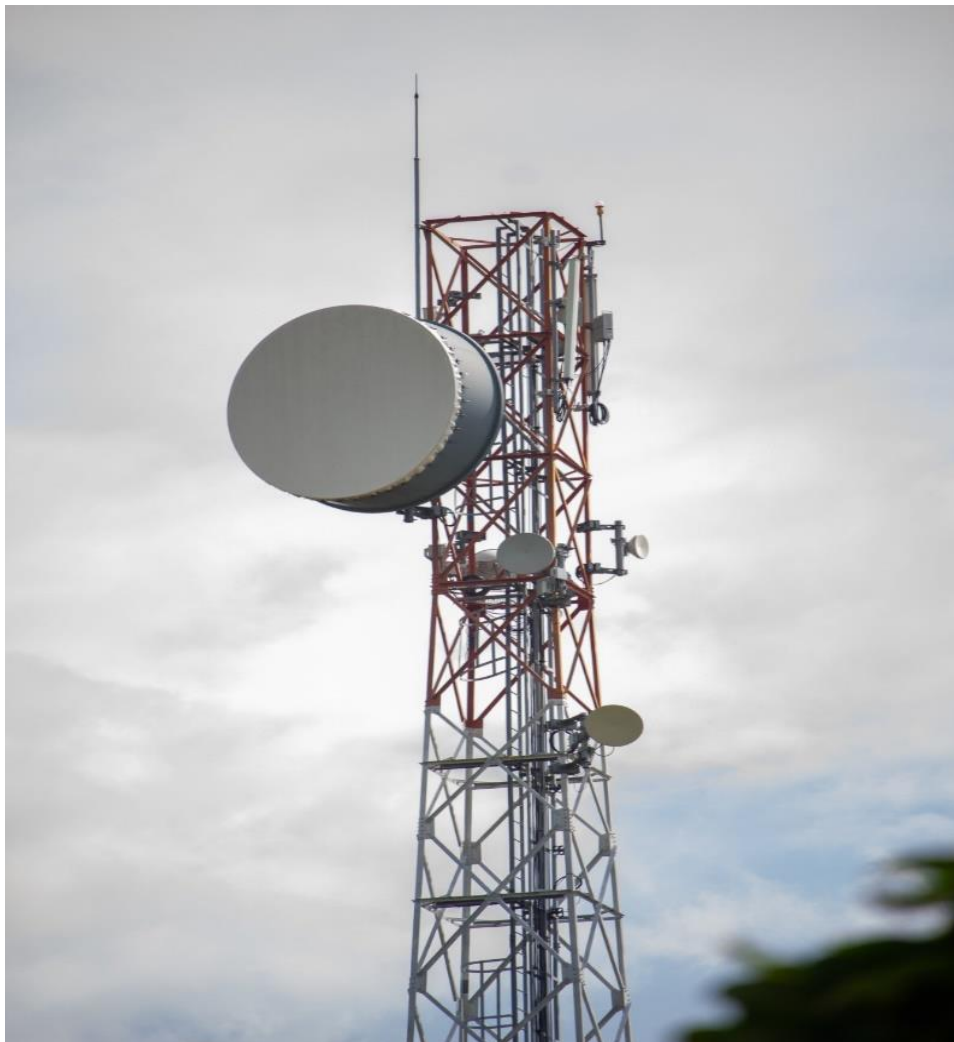
Figure 46. LPS for telecommunication tower
